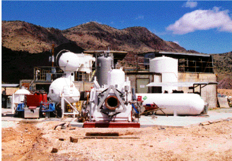
Figure 3. 80,000-lb. Thrust Engine Test Stand at the Energetic Materials Research Test Center (EMRTC) Rocket Test Site at Socorro, NM. The facility will be used to test the Microcosm 5,000-lb., 20,000-lb., 40,000-lb., and 80,000-lb. thrust engines.
